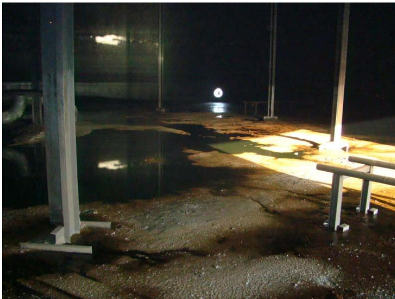
They described the results they achieved as "amazing"....they had cleaned down to the floor. Only hand lines were needed to finish the water wash. Asphalt is very hard to refluidize once it "cools/solidifies/crystallizes", and they had expected to have to do much more manual cleaning once the recirculation with the Twisters was finished.
